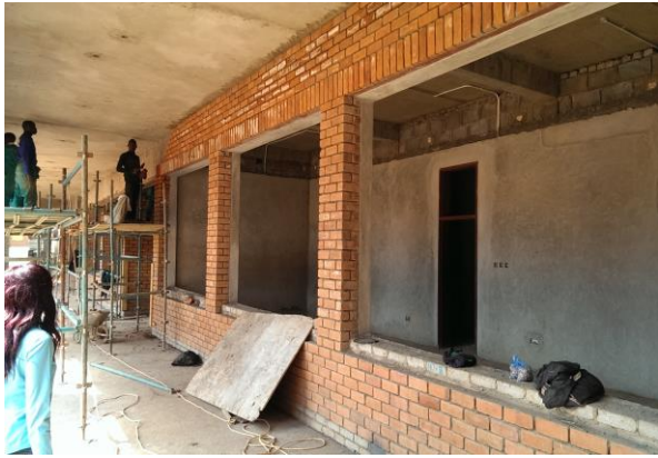
Figure 17: Infill walls of ground floor and internal plastering
