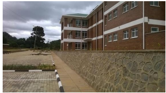
Figure 5: Completed side view of the hostel
