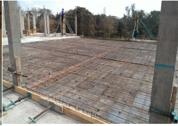
Figure 18: Main laboratory ready for concrete plastering
