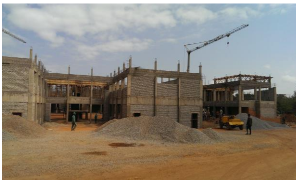
Figure 15: Group floor eastern wing external cladding in progress.
