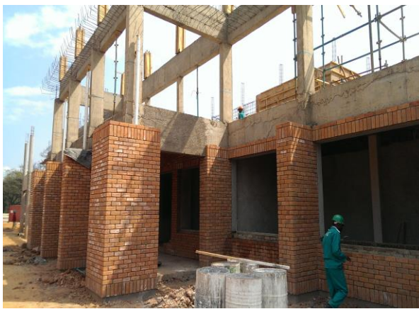
Figure 19: External cladding facing bricks
