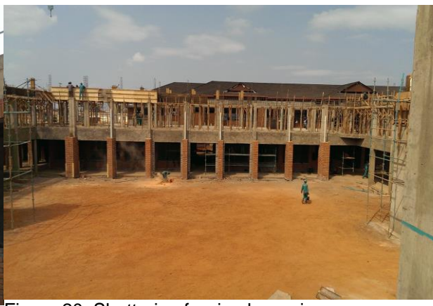
Figure 20: Shuttering for ring beam in progress
