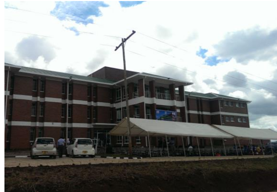
Figure 3: view of the hostel on official opening
