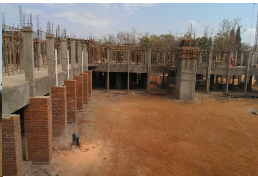
Figure 16: Lift well, external cladding and first floor columns to receive ring beam casted
