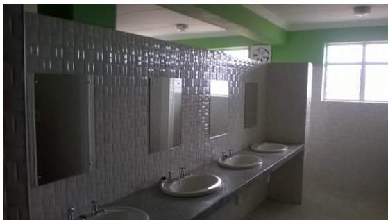
Figure 6: view of completed ablution areas
