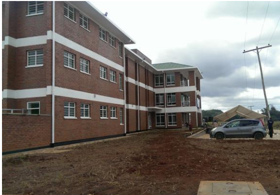
Figure 2: Completed side view of the hostel
