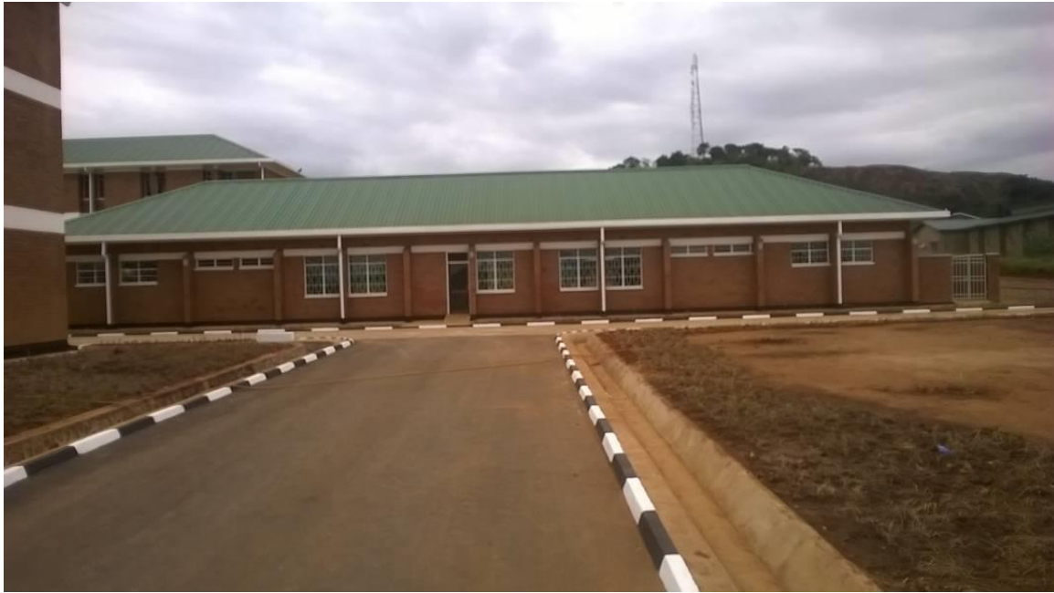
Figure 8: approach view of Completed Catering Block
