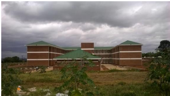
Figure 4: Completed rear view of the hostel
