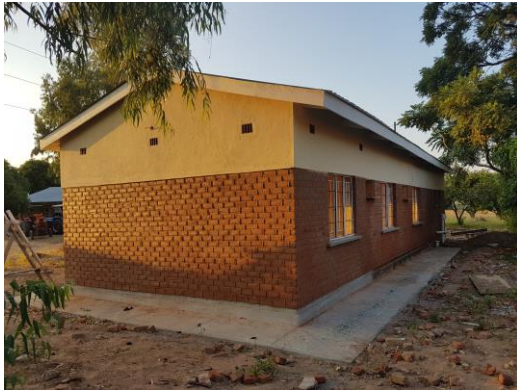
Figure 2: Building under renovation in Nkhotakota
