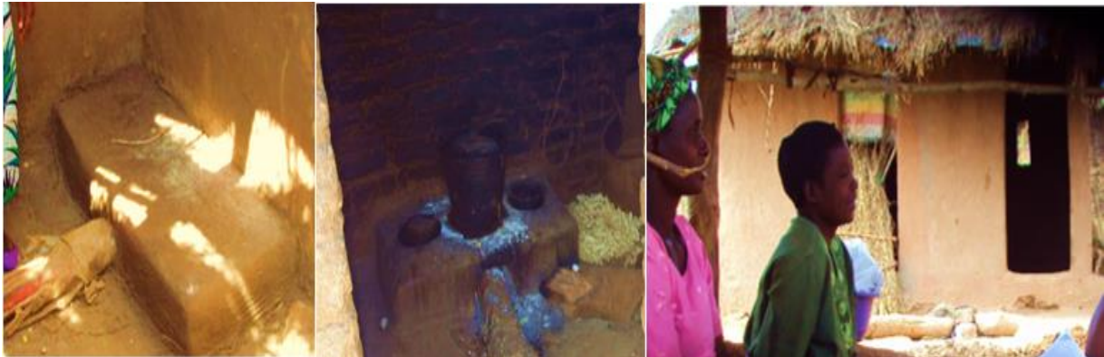
Photo 6.4: Fixed ICS leans on two sides, and one side of kitchen walls (left), small kitchen (right)
