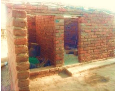
Photo 7.11: Newly constructed kitchen (Chisoni, June 2016b)
