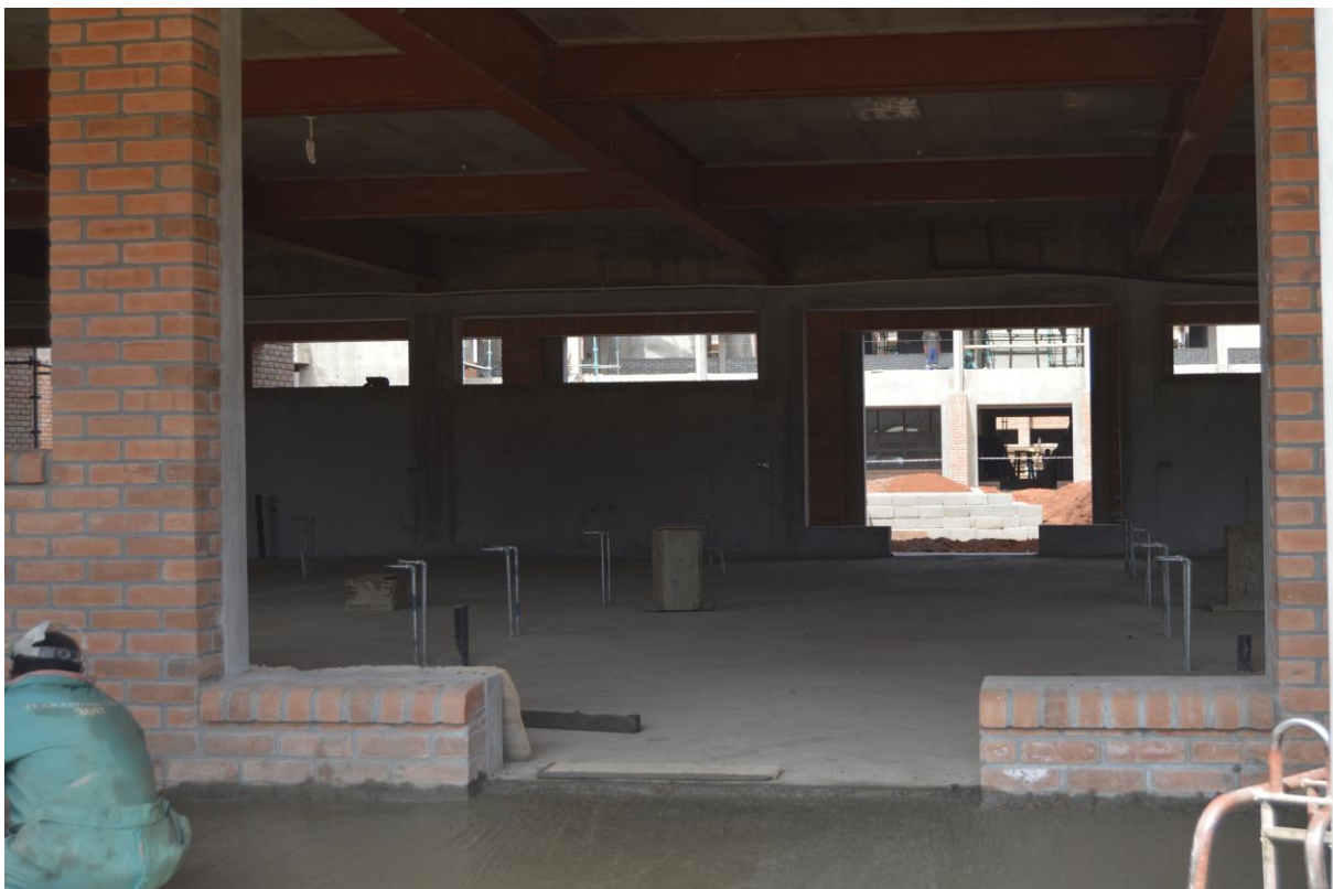
Figure 3: Installation of floor finishes
