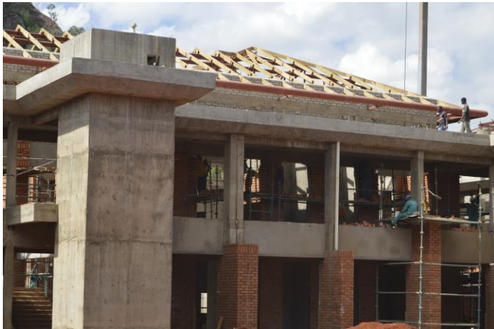
Figure 1: Construction of lift walls, roof rafters and purlins, veranda flat roof and external cladding
