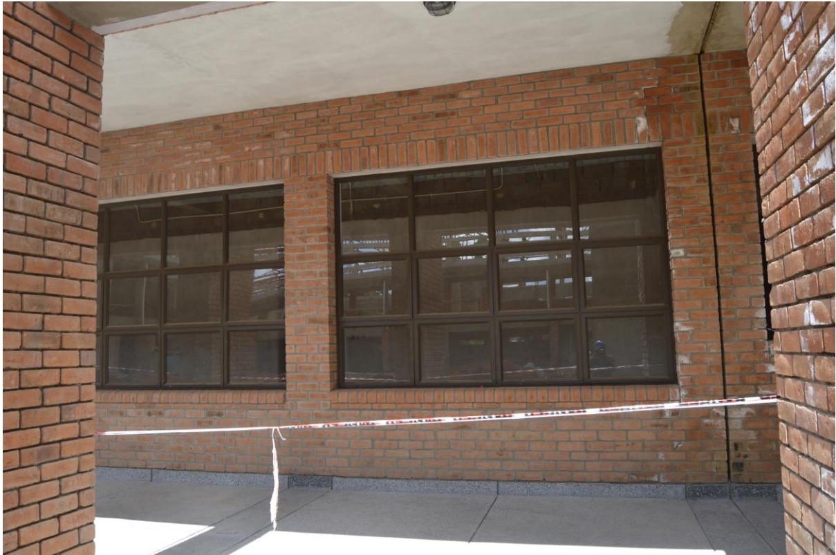
Figure 2: Installation of aluminium window frames and glazing
