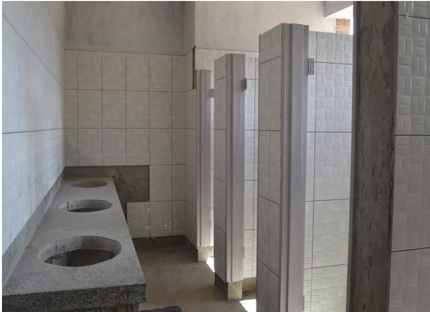
Figure 4: Installation of wall tiles, internal plaster and joinery in toilets
